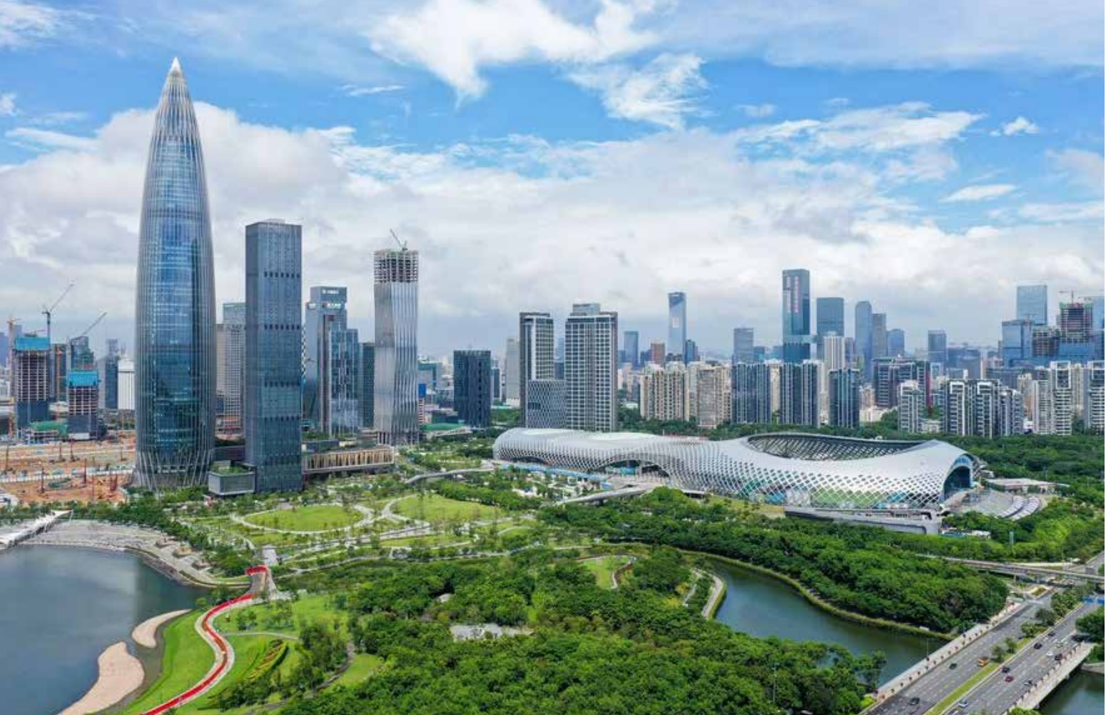
An aerial view of Houhai in Nanshan District of Shenzhen, in south China's Guangdong Province on Sept. 17, 2020.
