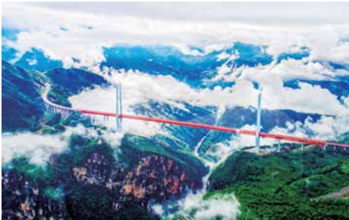
On December 29, 2016, Beipan River Oversize Highway Bridge was opened to traffic. With a full length of 1341.4 meters, a maximum span of 290 meters and a vertical height of 565 meters from the bridge deck to the valley floor, it became one of the prestressed concrete rigid frame bridges with the longest span in Asia. The drive from Xuanwei city in Yunnan province to Liupanshui city in Guizhou province is now shortened from five hours to one hour only. The picture shows the magnificent Beipan River Oversize Highway Bridge.
