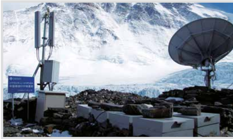
On November 13, 2007, China set up on EBC (Everest Base Camp) the highest-altitude (6500 meters high) 4G-base station of the world, with signals covering as high as the 8300-meter camp and its neighboring areas. By now, China already built up the largest-scale 4G network of the world, with 3.46 million base stations, covering all the urban and rural areas. The picture shows the highest-altitude (6500 meters high) 4G-base station of the world on EBC (Everest Base Camp).
