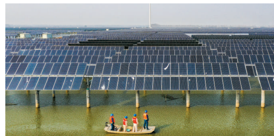
China has been boosting green development by promoting clean energy in recent years. Electricity workers patrolling amid a photovoltaic and wind power generation project installed above the fishery waters in Baoying County of Yangzhou, Jiangsu Province. (PHOTO: XINHUA)
