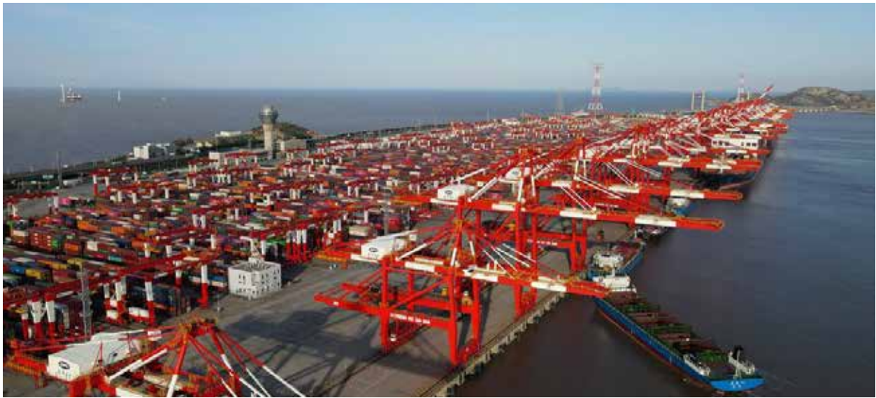
A view of the automated container terminal of Shanghai's Yangshan Port in east China.
