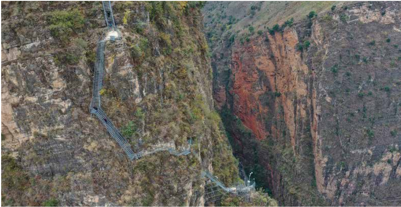
A steel ladder built on the cliff in Atulieer Village, Zhaojue County, Liangshan Yi Autonomous Prefecture, southwest China's Sichuan Province.
